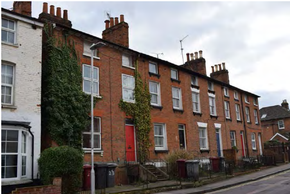
Figure 6.3.13 23- 31 Baker Street, Alexandra Terrace, c.1850, red brick terrace, overall well-preserved with majority of original windows and doors intact
