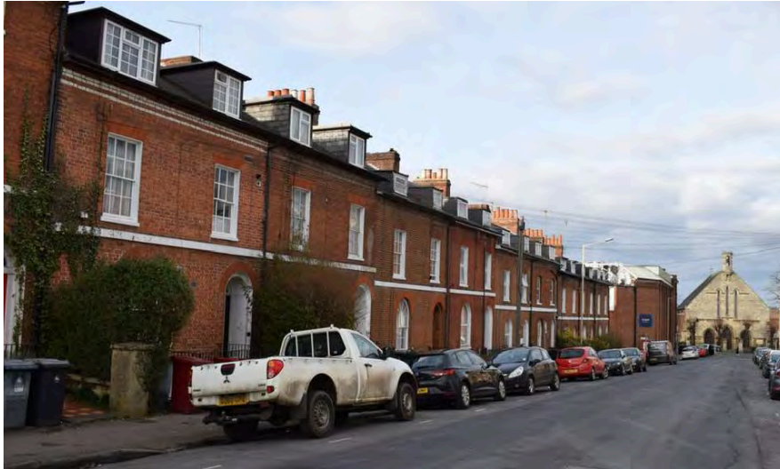
Figure 6.3.7 Georgian terraces at nos. 6-14 Russell Street. The Holy Trinity parish church forms an impressive view at the north end of the street from the Oxford Road
