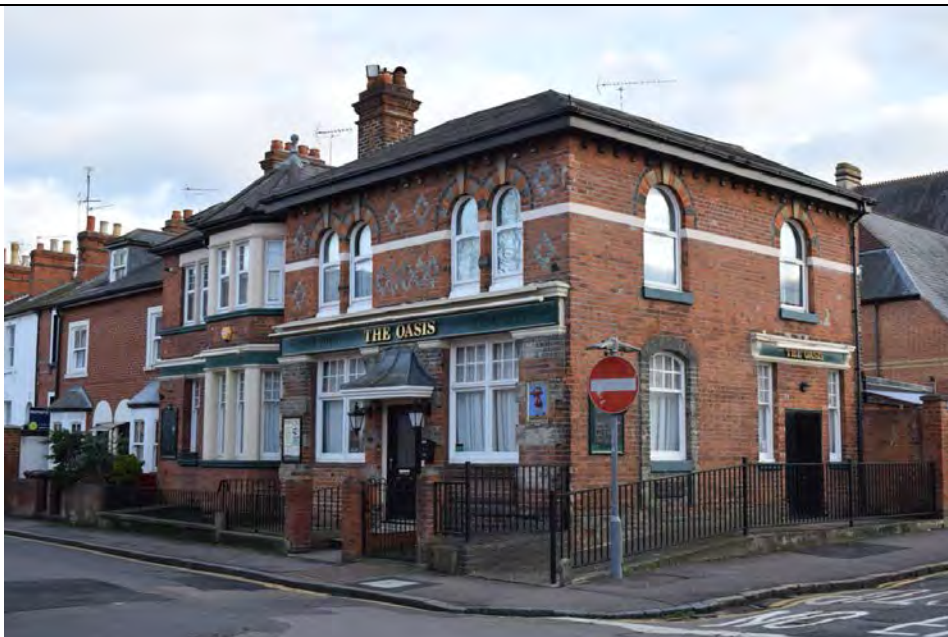
Figure 6.3.15 The Oasis Community Centre, c.1860s Inn and Public House
