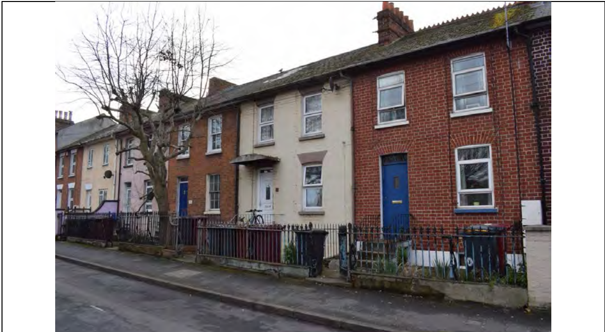
Figure 6.3.5 Original iron railings at 16-22 Howard Street and the curved stucco dividing wall at no. 22
