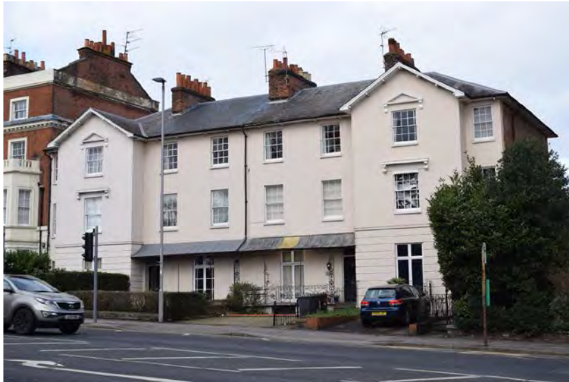
Figure 6.1.16 Nos. 162A-168, with Regency iron detailing, an early Jesse family development
