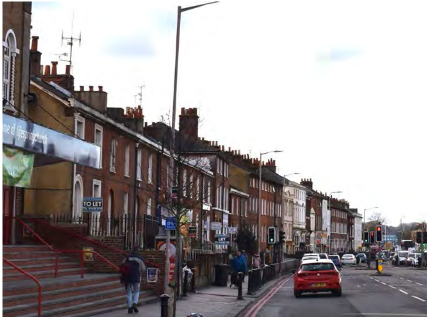
Figure 6.2.7 Listed Georgian terraces along Oxford Road, in poor repair, lost behind cluttered street furniture and busy road traffic
