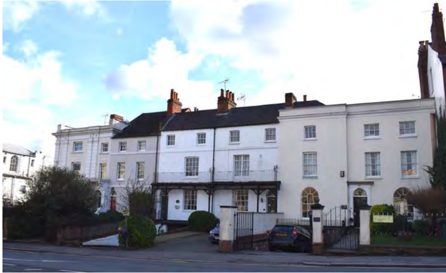
Figure 6.1.14 Attractive diverse terrace of Georgian properties at 113-121 Castle Street
