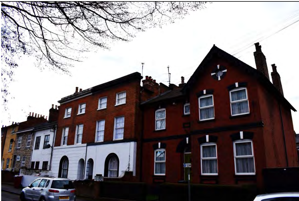
Figure 6.3.4 2, 4 and 4A (listed Georgian semi-detached) Howard Street showing the rustication on 4A
