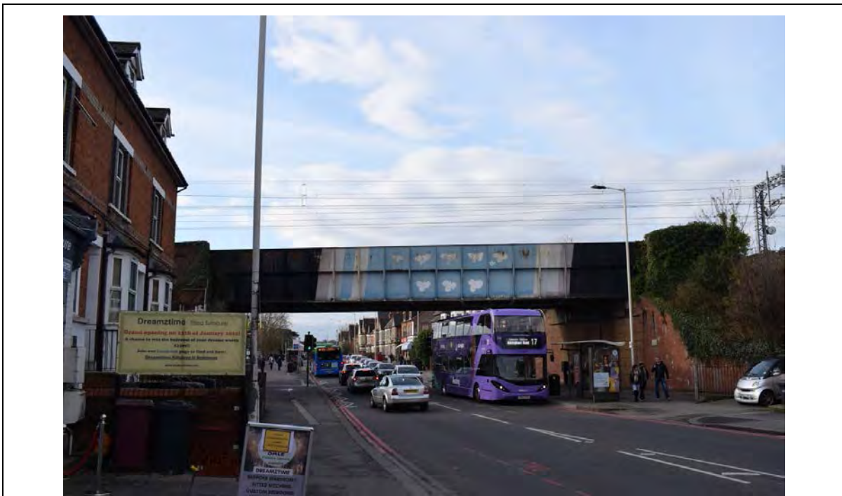
Figure 6.2.2 Reading West railway bridge, facing west along the Oxford Road, the iron bridge replaced an original brick design
