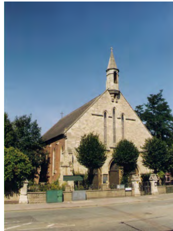
Figure 6.2.11 Holy Trinity spiralet before removal
