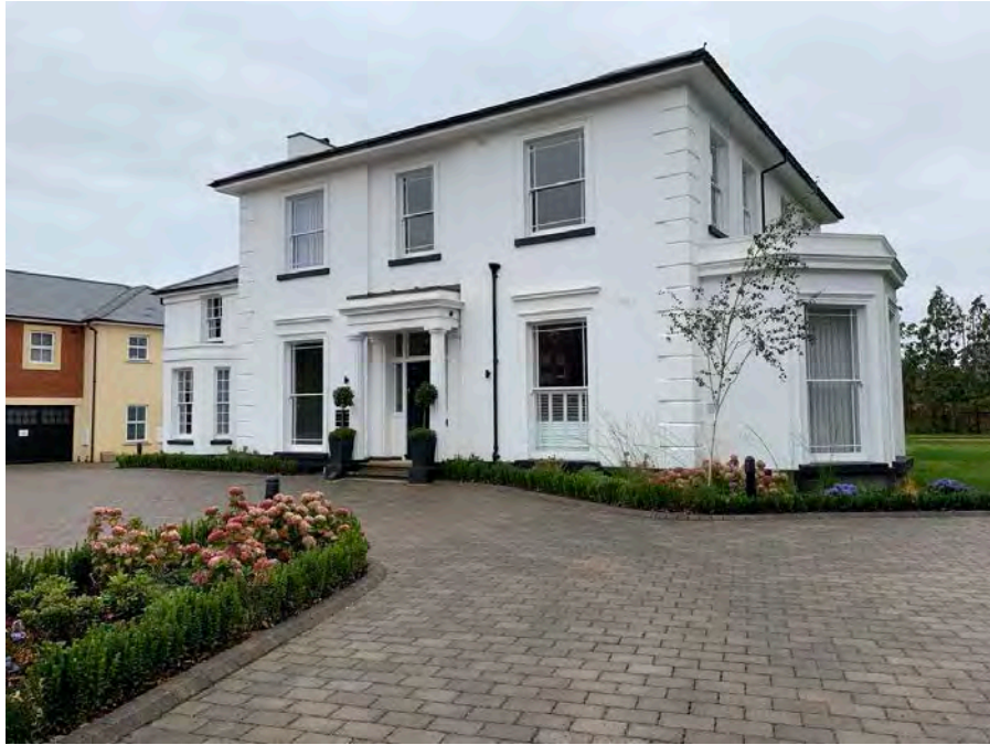
Figure 6.5.5 3 Castle Crescent after recent renovations
