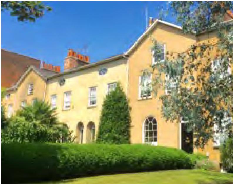
Figure 6.1.13 Bath stone coloured stuccoed Regency style terrace, 134-144 Castle Hill
