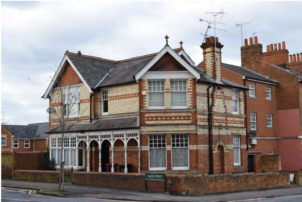
Figure 6.3.10 The Parsonage (c.1890) at the northeast corner of Baker Street and Russell Street with attractive polychrome and wood detailing
