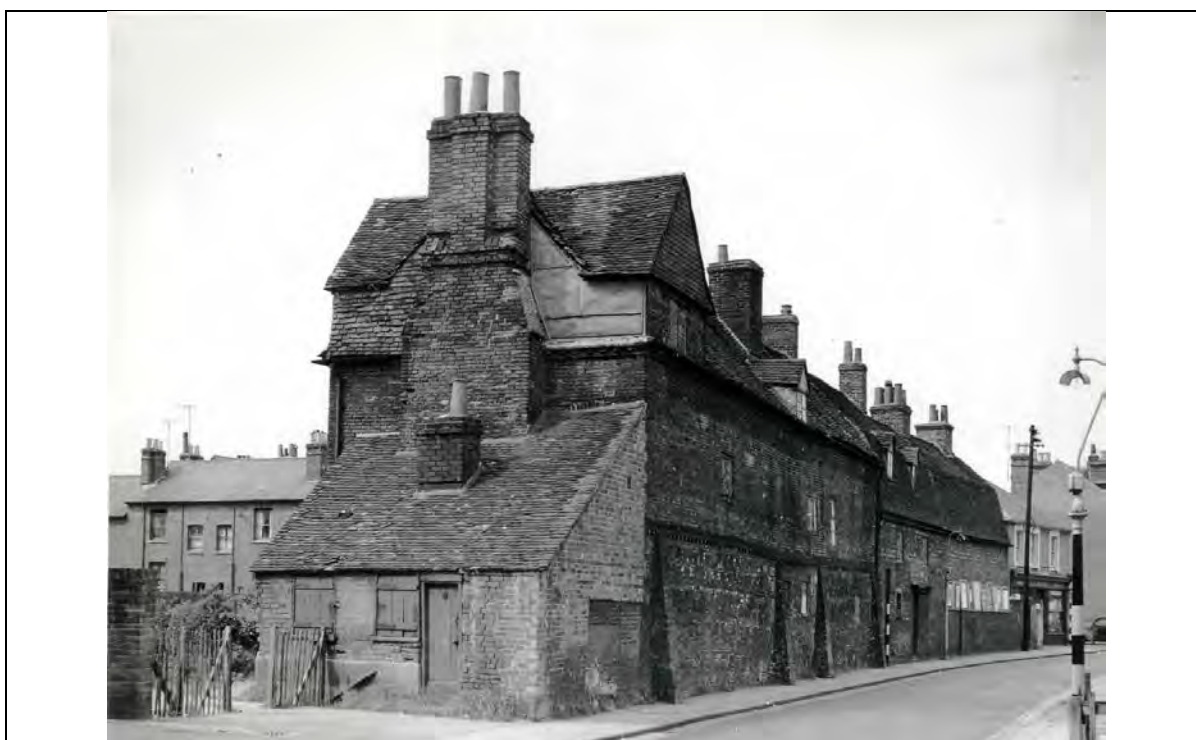
Figure A1.12 Finches Buildings- demolished for the IDR. The side of 3 Baker Street at the far right
