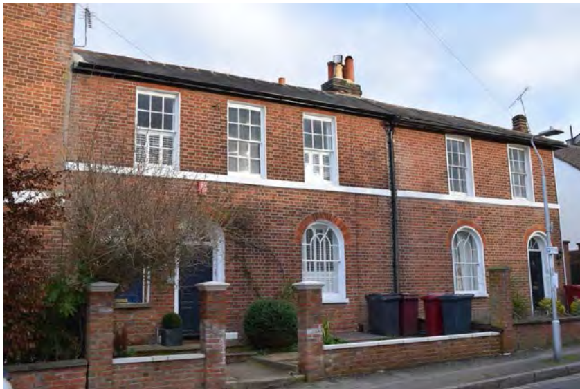
Figure 6.5.4 Arched windows and fanlights on two storey Georgian houses, Coley Hill
