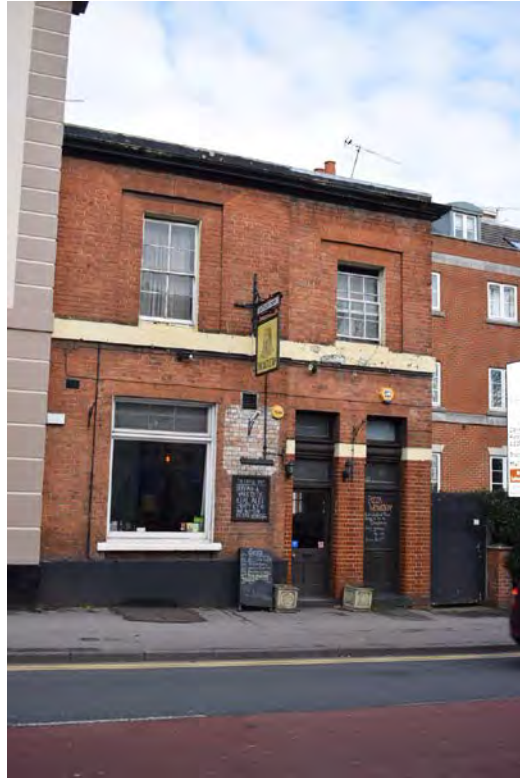
Figure 6.1.5 The former Horse and Jockey (The Castle Tap) rebuilt early 19 th century, 120 Castle Street
