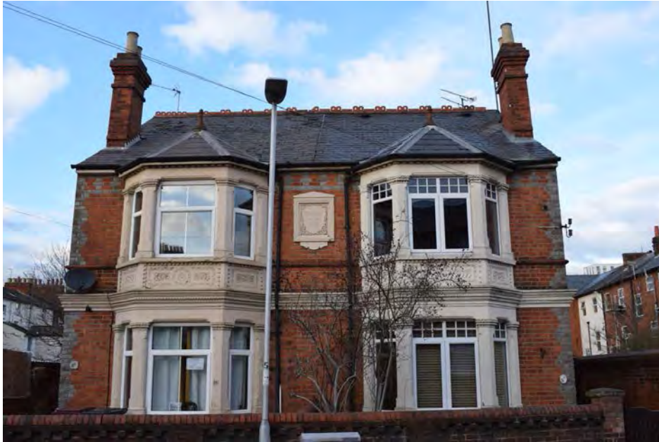
Figure 6.3.14 Rednirt Villas 1904, developed by Mr. Trinder, bay windows, polychrome and stone work detailing. Rednirt is Trinder spelt backwards.
