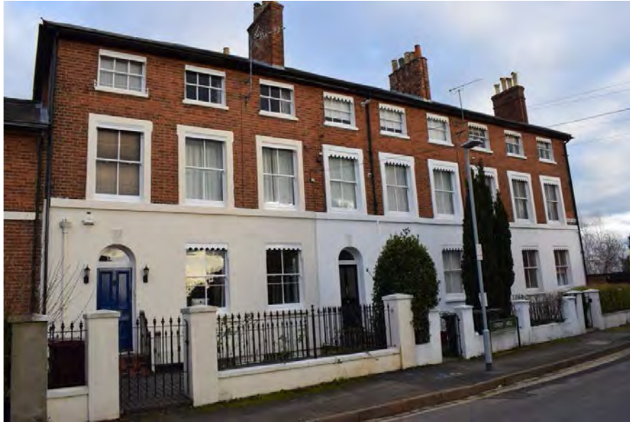
Figure 6.5.3 31-35 Coley Hill, stuccoed lower ground floor and later Victorian trimmed windows, 1820-30s
