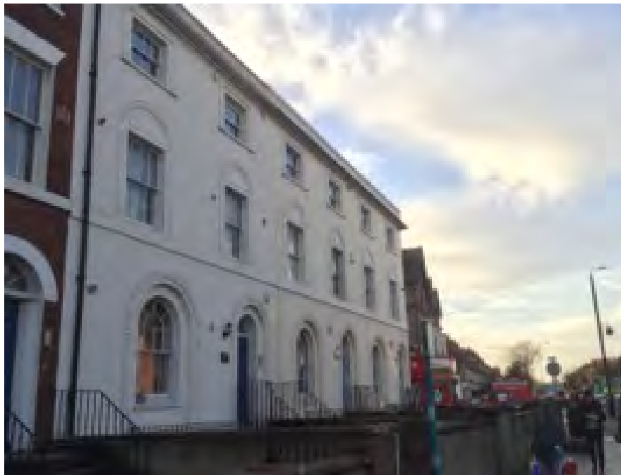
Figure 6.2.4 Large stuccoed Georgian Sidney Terrace, 197-203 Oxford Road
