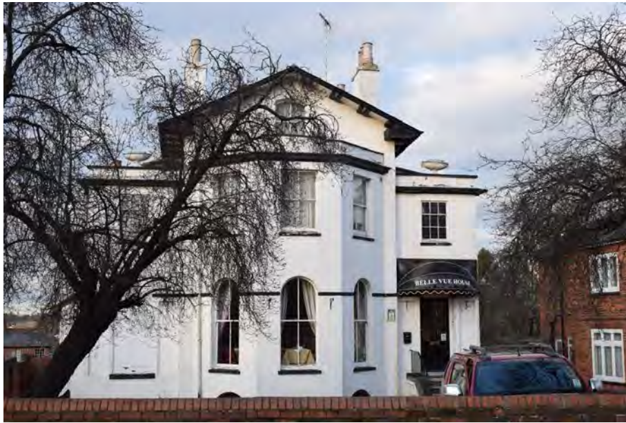
Figure 6.4.5 Bellevue House, 2 Tilehurst Road, built prior to 1839, listed, with decorative urns possibly of Coade stone.
