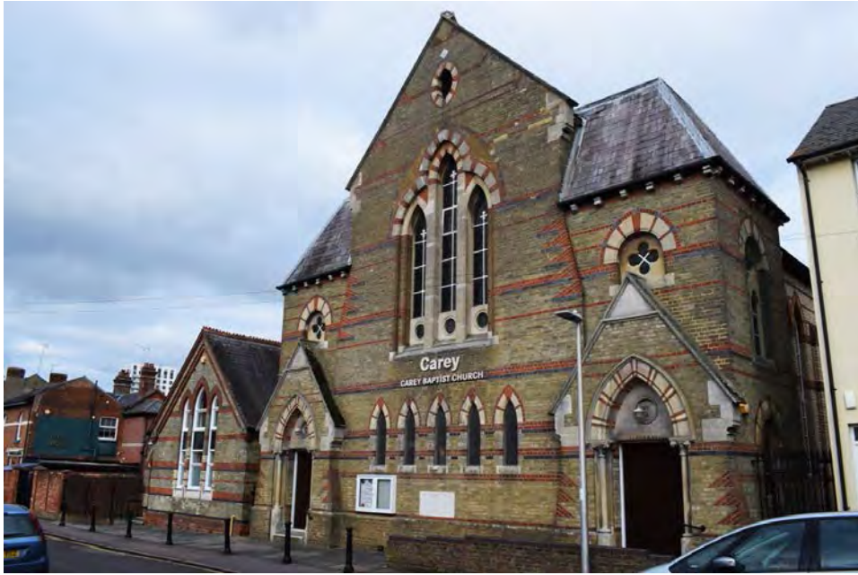
Figure 6.3.20 Carey Baptist Church chapel with its polychrome frontage, 1869
