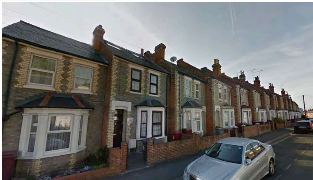
Figure 6.5.9 Field Road polychrome terrace
