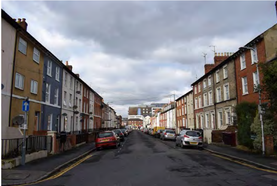
Figure 6.3.17 The conditions of terraced housing along Zinzan Street with poor quality modern dormers, overhead wires, excessive bins and satellite dishes.
