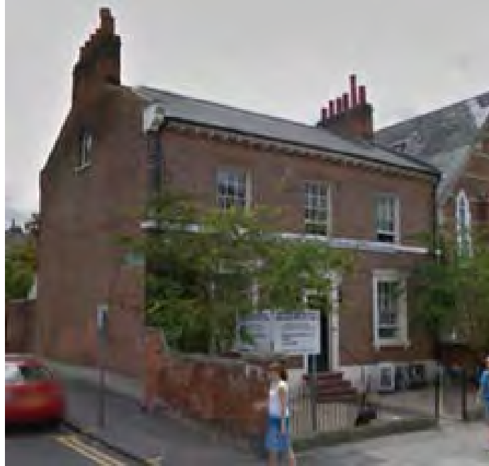
Figure 6.2.5 101 Oxford Road-a detached Georgian family home with original high back garden walls
