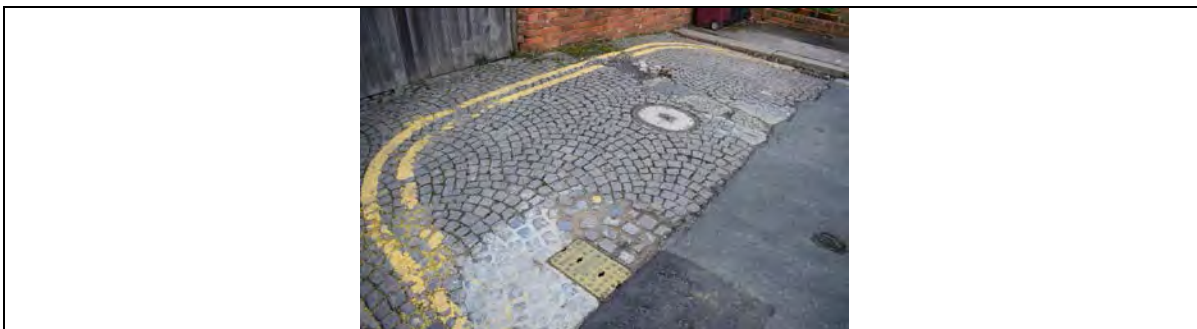
Figure 5.5.3 Sett stone pavement at the end of Belle Vue Road, still displaying the fan pattern of road that was common in the area.
