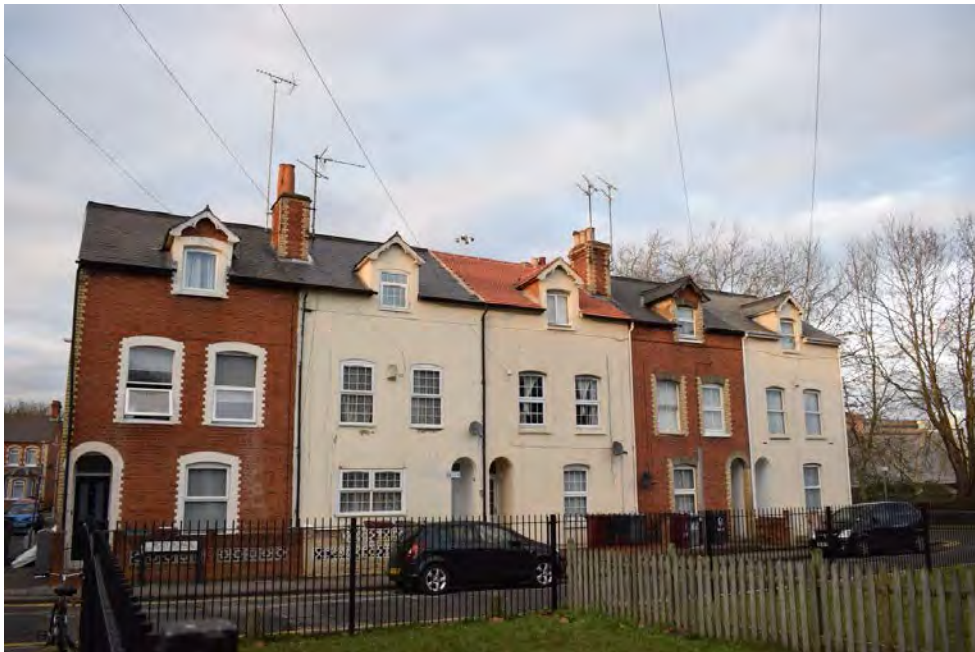
Figure 6.3.21 6-12 Body Road, the new red tile roof was installed during the time protection of a Conservation Area did not apply, after 2004
